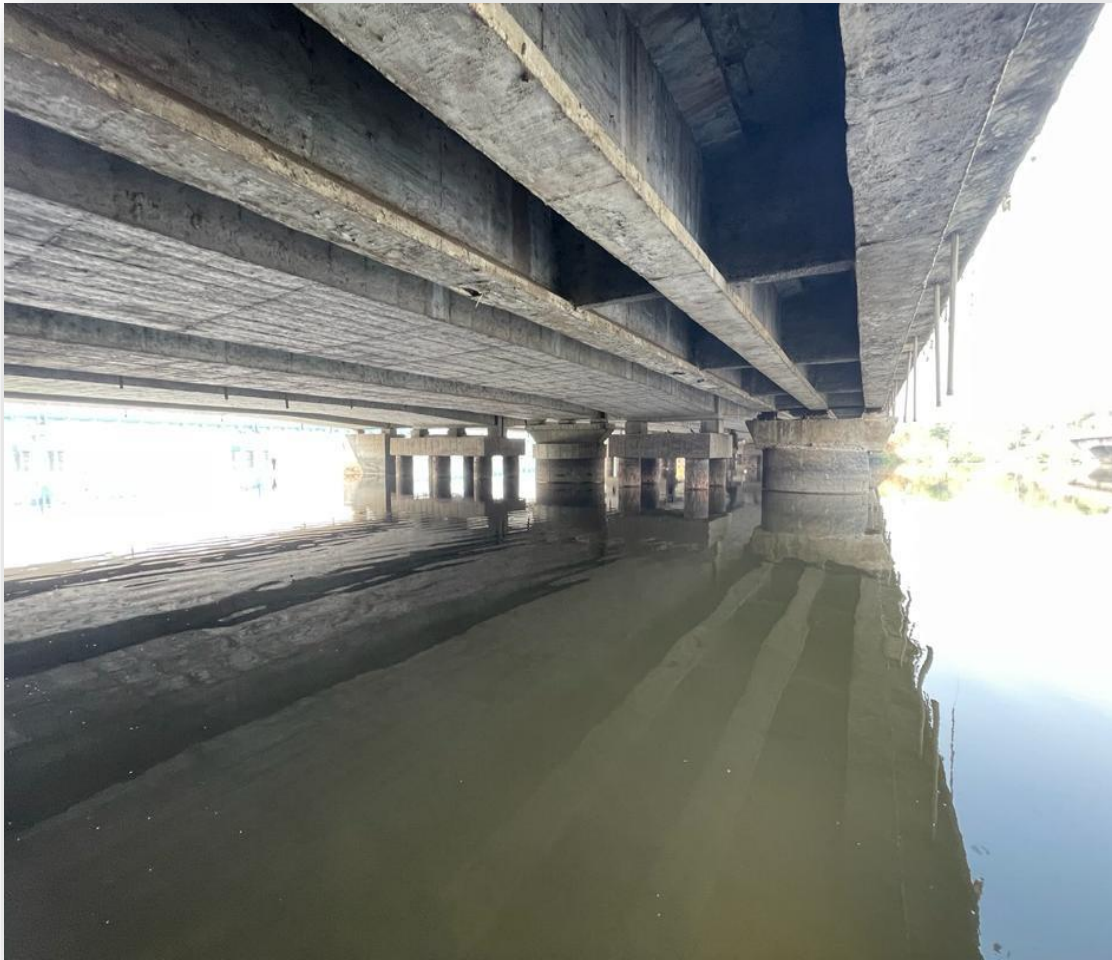
Reconstruction of Taloja Creek Bridge, Raigad
