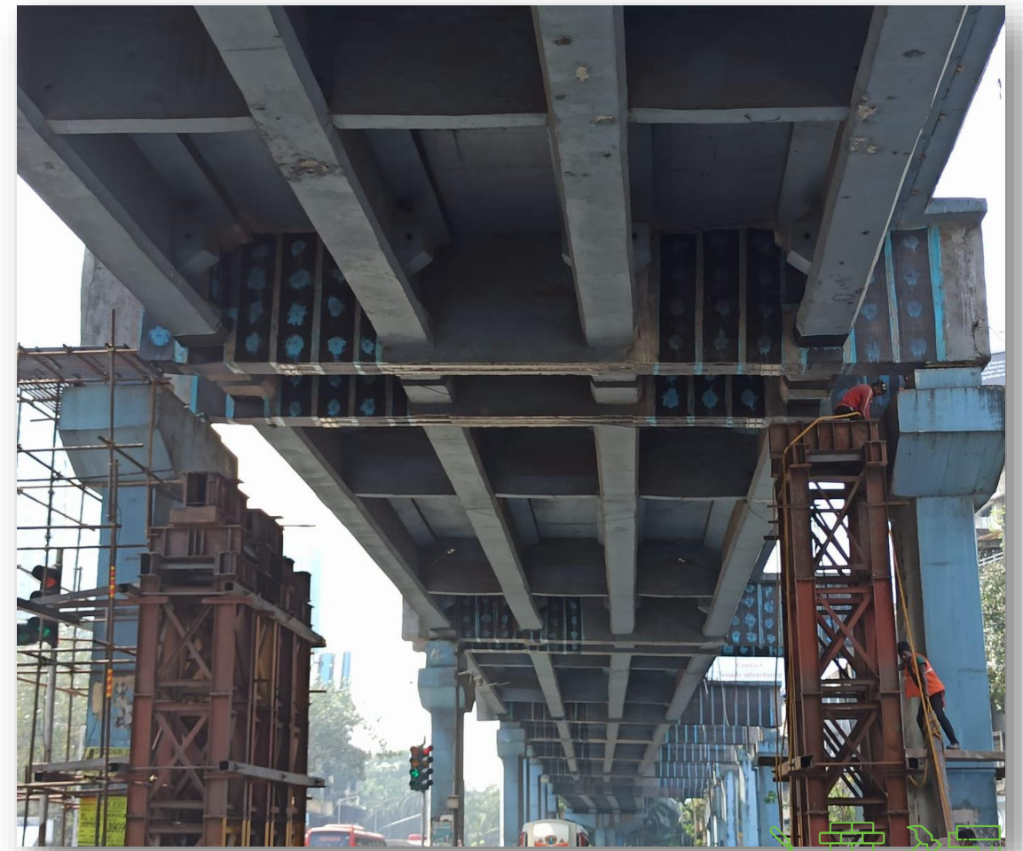
Retrofitting & Repairs of Bridges in Mumbai
